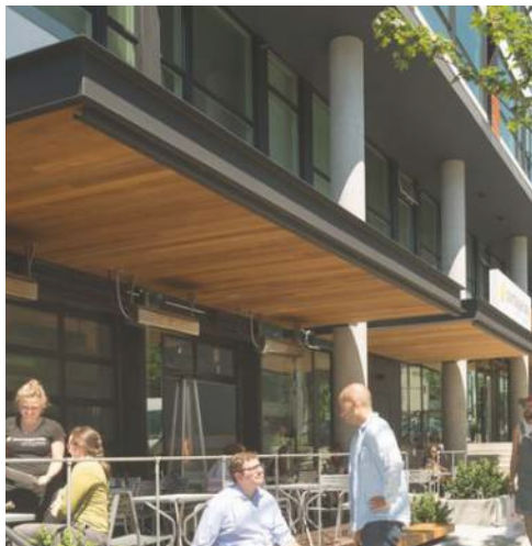
Exterior Fixed Canopy Aluminum frame with solid infill
